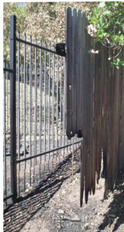
Undamaged metal fence next to a burned wooden fence
