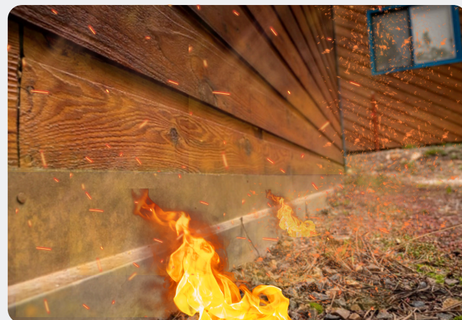
Metal flashing helps prevent debris from igniting wood siding
